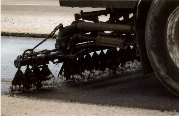
Top: Preparing for new pavement inlay at SH 64.
