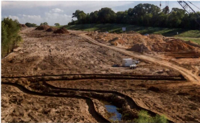
Top: Conducting earthwork.
